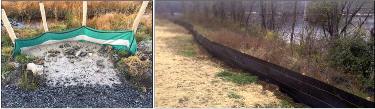
Figure 8.2: Silt fencing measures (Source: Hy-Tex (UK) Ltd. (left) and Thrace Group (right))
